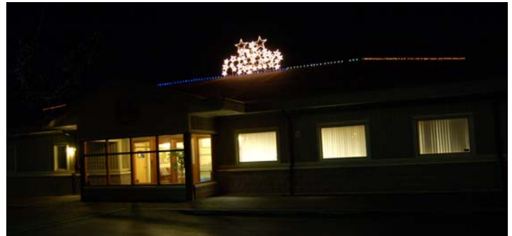
Roof Top Display
